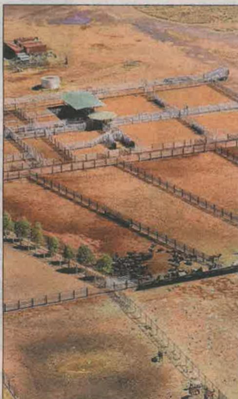
MASSIVE YARDS: Balfour Downs famously features 3000 head capacity steel cattle yards.
